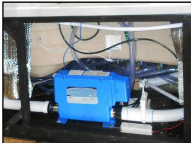
Pictured above is the inside of the spa behind the front door. The electrician now has access to connect the spa for power. While the front door is off, refer to page 12 for instructions on ensuring the plumbing fittings are secure (but do not be tempted to over-torque or over-tighten these fittings).
