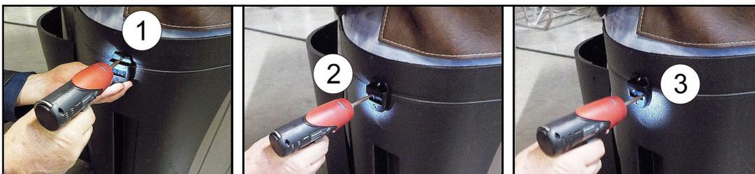
**Step 4.** Use a screwdriver to finish screwing in the 3 screws. (Repeat this process for the other 3 corners.)
